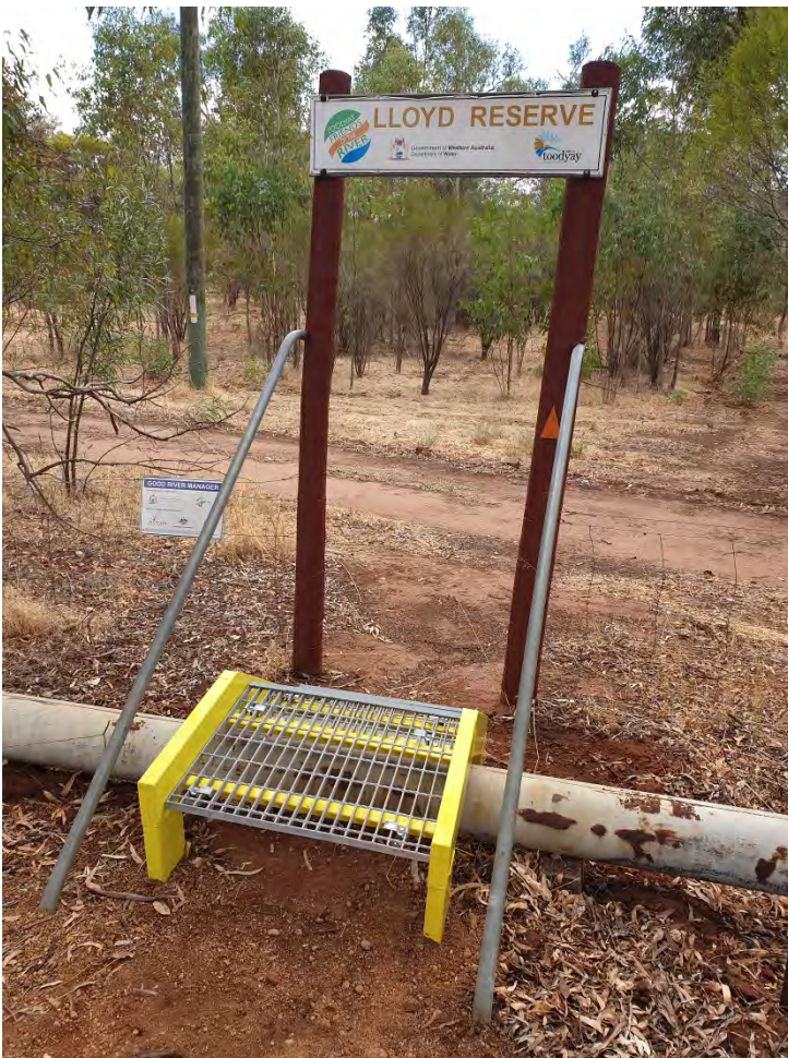
Left: The recently installed steel fabricated step over the water pipeline.
